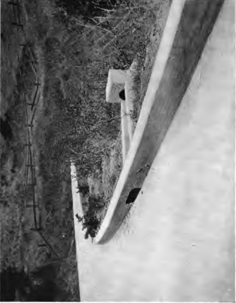
This picture shows in detail the poured curbs used in State Highway work. Corrugated pipe spillway carries off water, preventing bank erosion.
